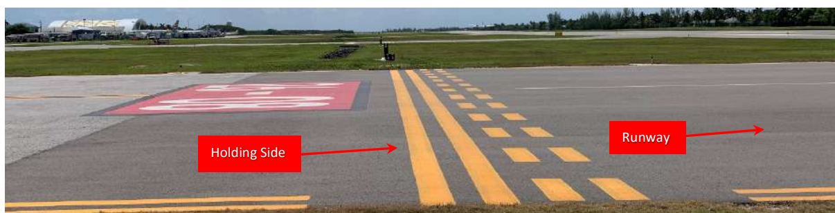
Figure 9 – Runway Holding Point
