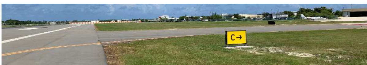
Figure 11 – Runway Exit Sign
