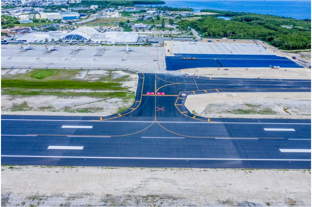
PHOTO 2 SUBMITTED: New junction of Taxiway Foxtrot and Taxiway Gulf
