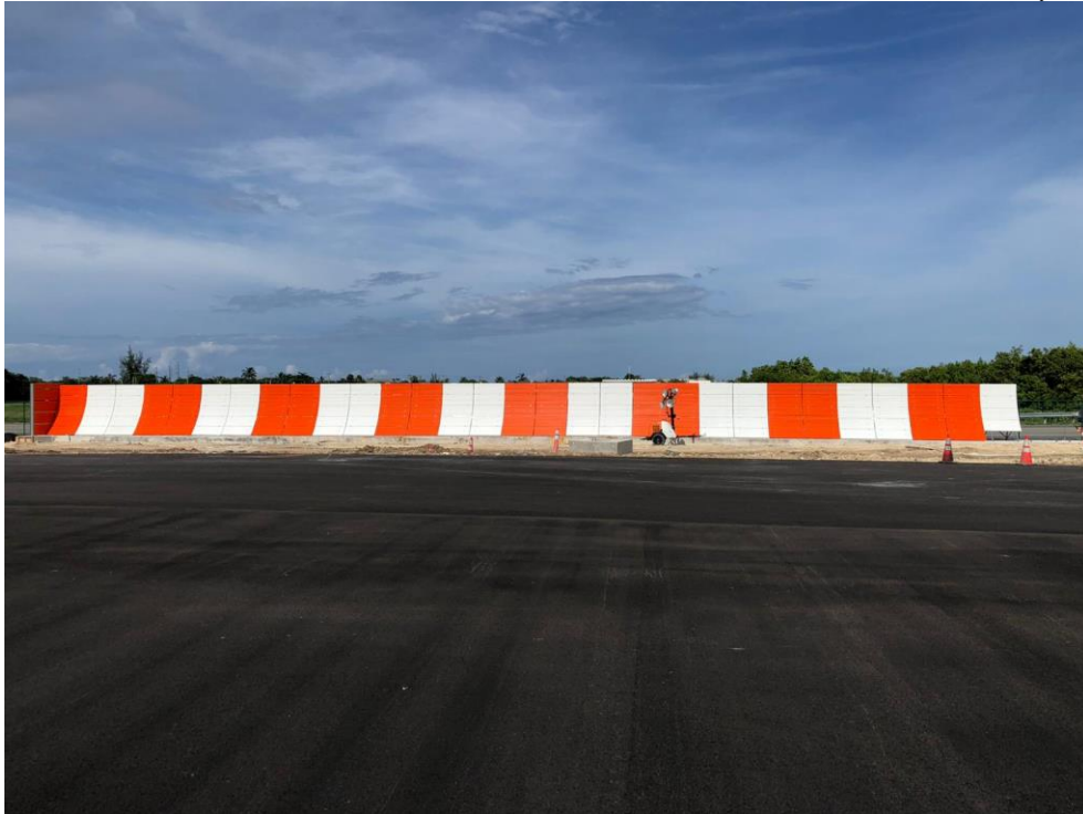
PHOTO 1 SUBMITTED Cayman Airport Gets New Aircraft Jet Blast Deflector: A section of the new blast deflector at Owen Roberts International Airport.
